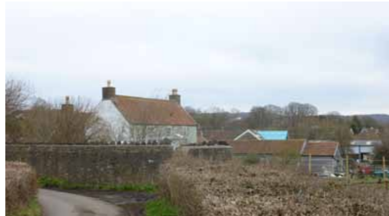
Coombe Grange Farmhouse (Grade II Listed Building)
