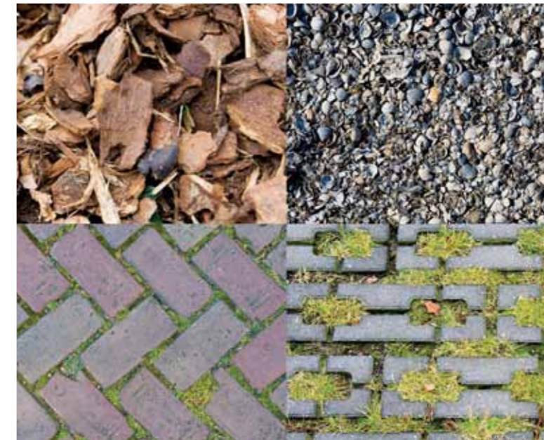
Permeable surfaces with cellular attenuation
