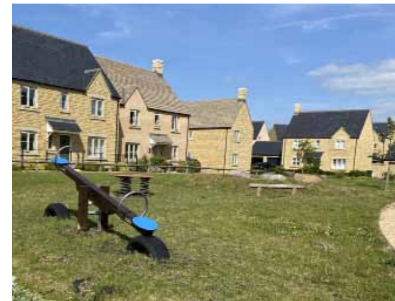
Housing in on the edges of the site with shared surface for access to individual properties
